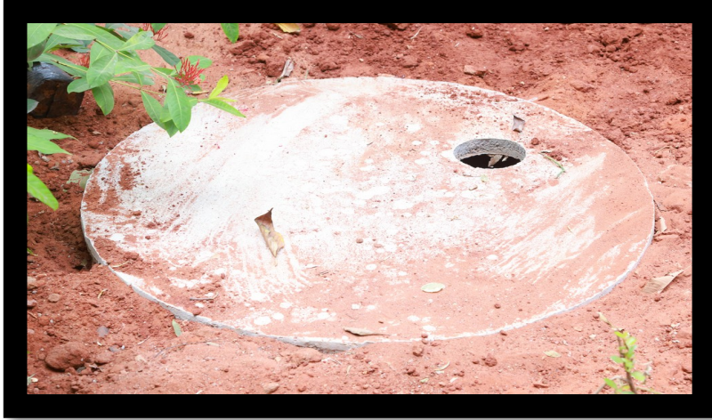
Rain water harvesting pits
